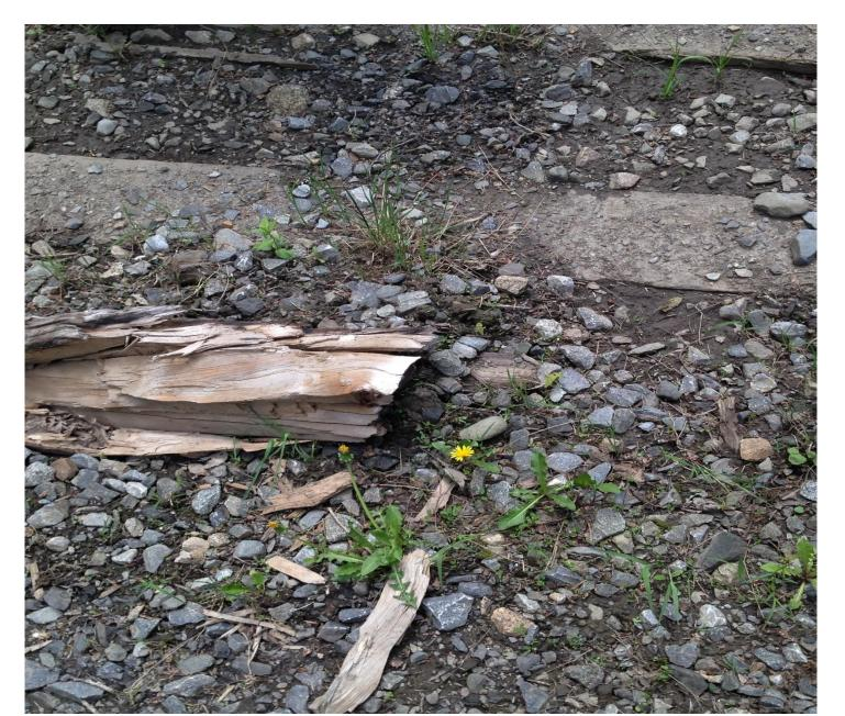
Vegetation, sunken ties, poor drainage→ mud build up in rail bed Runoff ditch with scummy water off edge of ties
